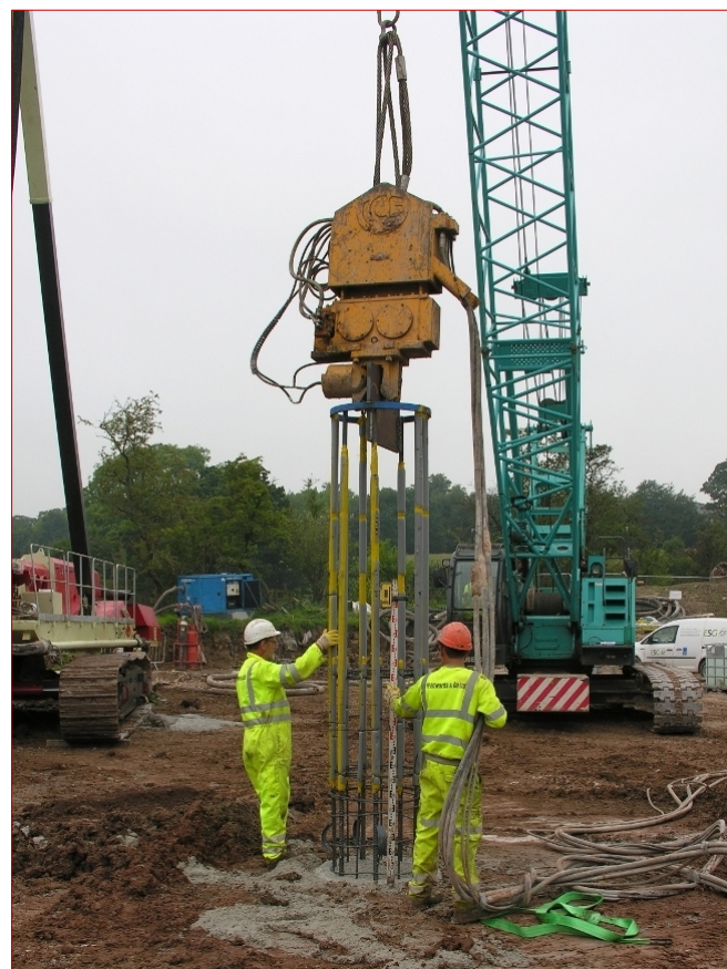
Reinforcement cage insertion by vibrator
