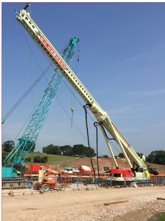
Rigging of the Llamada P240TT
