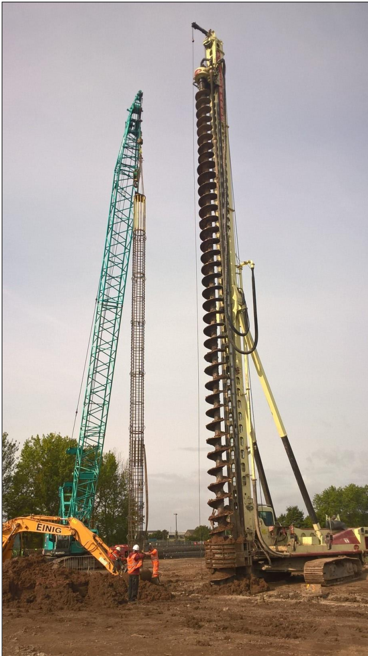
Llamada P135 installing 1050mm diameter CFA piles reinforced with 23m long reinforcing cages
