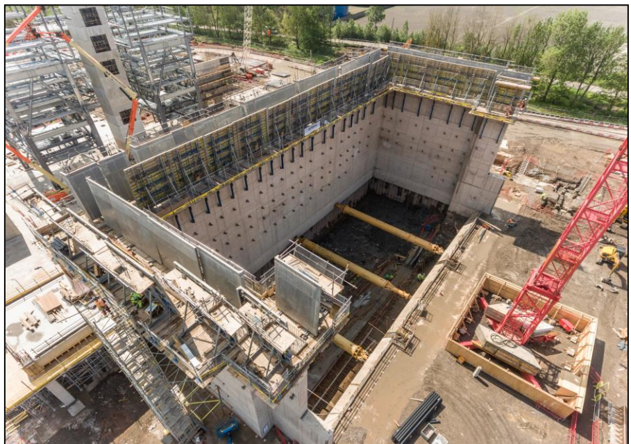
Waste bunker under construction
