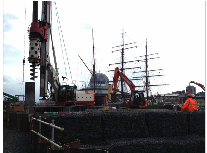
Piling adjacent to the RRS Discovery
