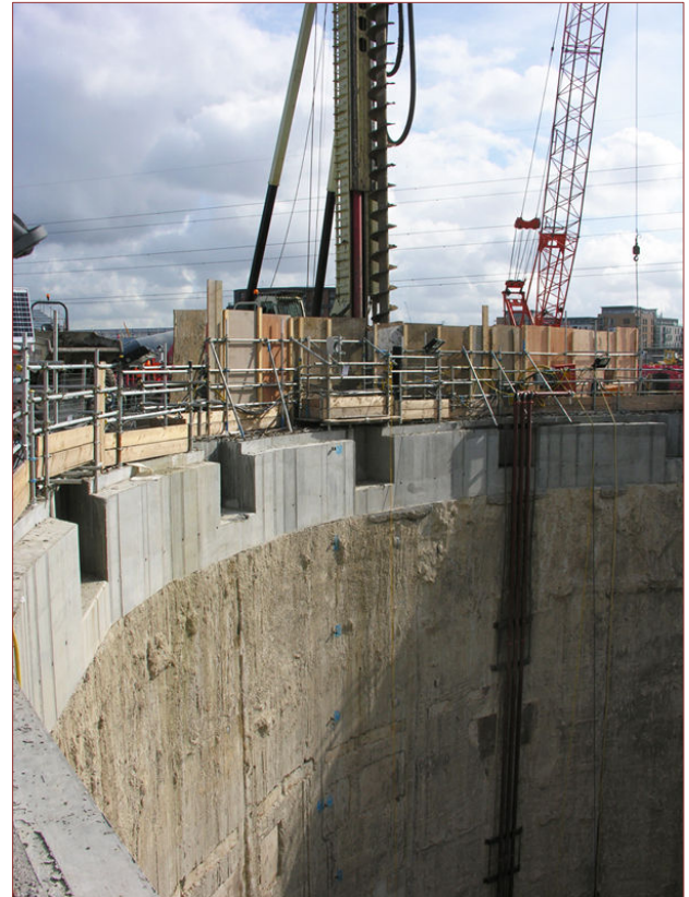
CFA piling in very close proximity to the Diaphragm Walled Shaft
