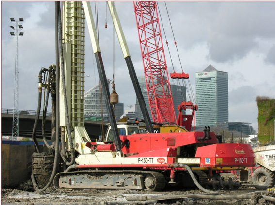
The Llamada P-150tt Rig used for the Project
