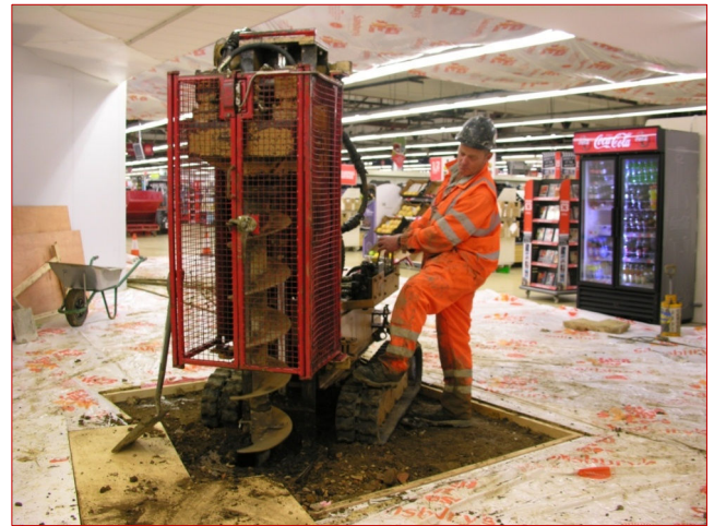
Technodrill TD308 installing mini piles at night in actual sales areas
